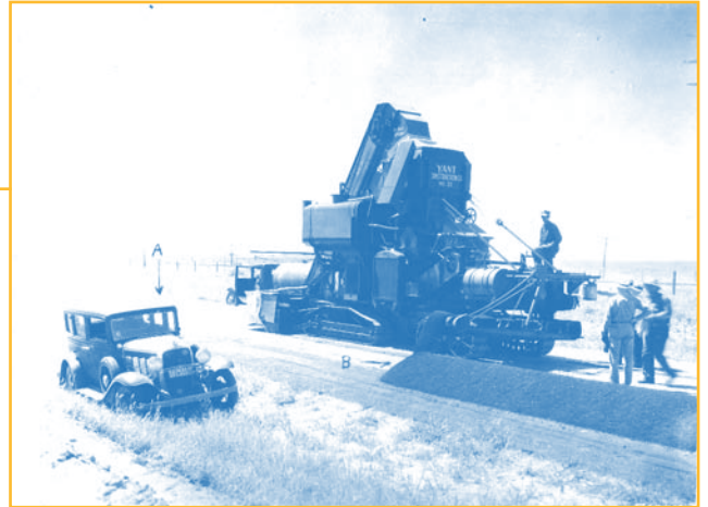
Barber-Greene Road Mixer on US 50 in Ohio. Courtesy: Asphalt Institute
